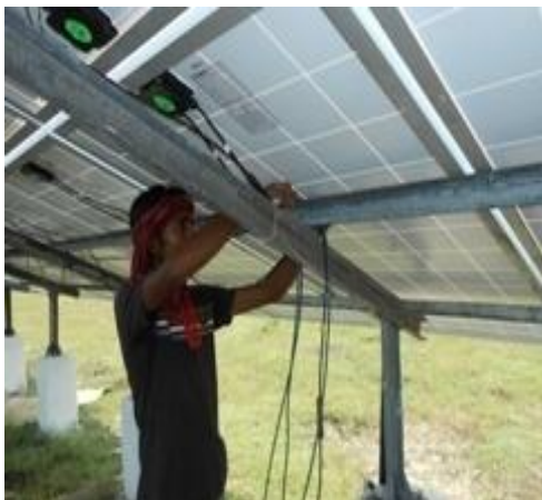
Plate: Cable connection
