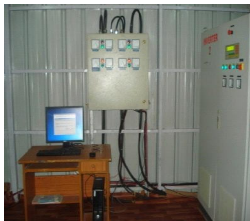
Plate: Computer system and DCDB box
